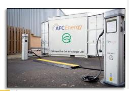
Alkaline fuel cell system development company, AFC Energy's H-Power works through a combination of HydroX-Cell(L)<sup>TM</sup> fuel cell and battery storage or supplementary grid power.
